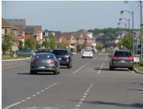
Figure 2.5 – Conventional Bicycle Lane, Milton Trails
